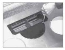
Place rectangular transition adaptor as shown by first installing 4 screws on half round section.
